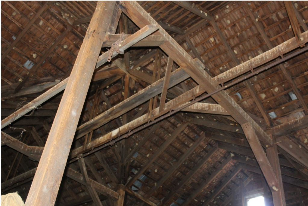
Photo 27: The open grain storage of the second floor retains its original hay trolley
