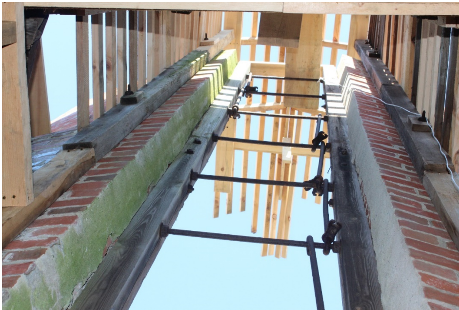
Photo 34: The continuous door slit of the silo runs along the south side of the silo.
