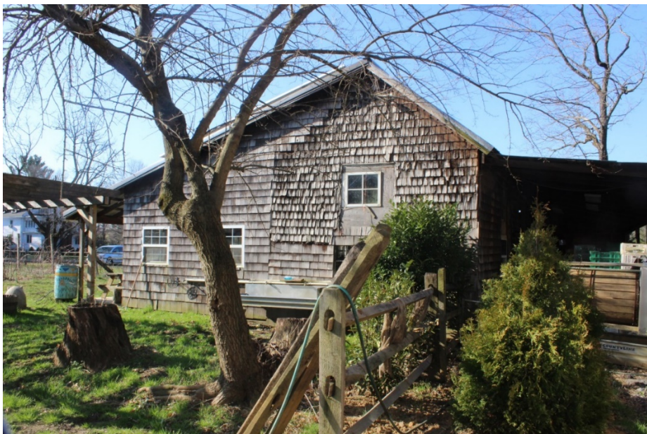
Photo 40: On the north elevation, the volume and roofline of the original 19 th century building is visible to the right with its older shingle cladding and 4-light wood window.
