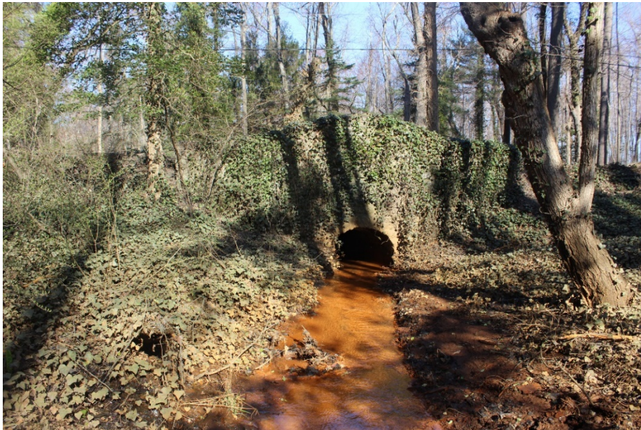
Photo 60: This stone culvert allows Fern Brook to cross under the north driveway. Looking north.
